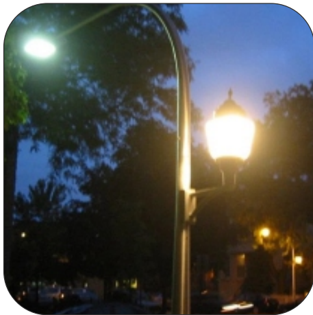
Metal Halide Street Lights
